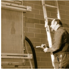
Masonry water penetration
