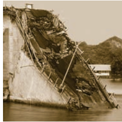
Palau bridge collapse
