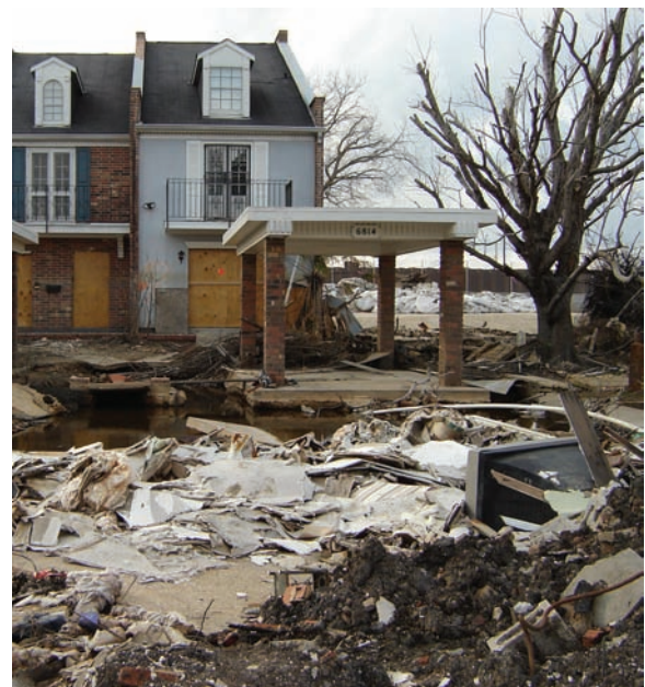
Damage assessment after hurricane Katrina.
