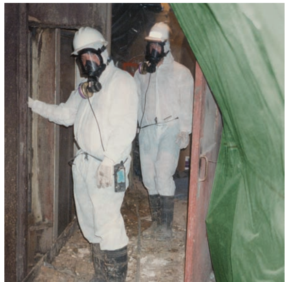
Asbestos removal inspection
